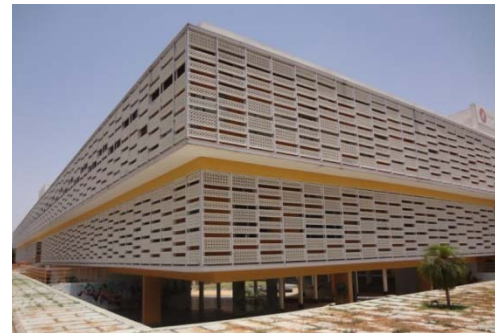
Fig. 26 : Double skin on Exterior by jali
