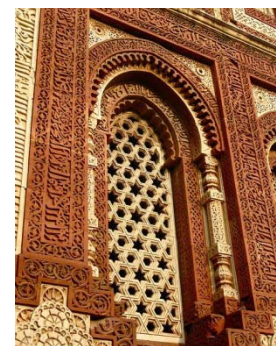
Fig. 17 lattice screen on façade
